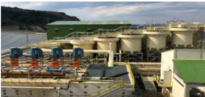
The Ivrandi ADR plant designed and built by KCA/DAMA Engineering in 2019, incorporating adsorption (CIC), acid washing, carbon stripping and generation, electro-recovery, mercury retorting and gold smelting units. It is one of Europe's highest capacity gold recovery plant with a 7 tons carbon capacity.
